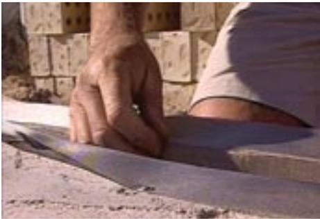
Stainless steel mesh systems incorporate finely woven, high grade stainless steel mesh. This can be used in the same manner as the traditional ant cap, being placed under the entire concrete slab area, around the perimeter of the building as a partial barrier or around individual penetrations. Combinations of physical and chemical systems may be necessary in some instances.
