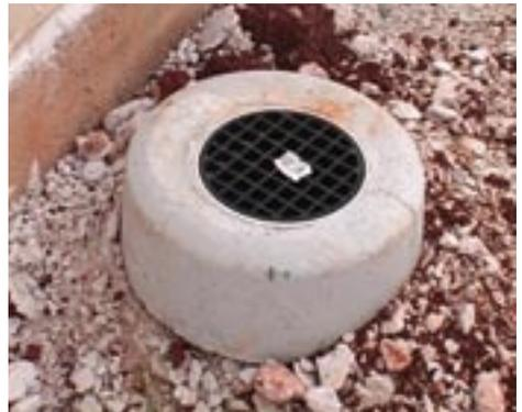
The installation of concrete protection blocks over exposed pipework and at inspection points and the like can provide an easy point for concealed entry of termites unless adequate measures are taken. In the case of chemical perimeter systems, these protection blocks need to be placed in position after the system has been installed, being careful not to disturb the system.
