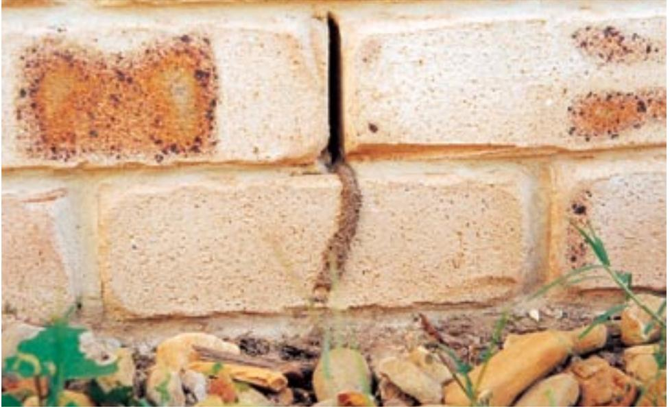
Regardless of the system used, regular inspections should be carried out by a BSA licensed contractor with the appropriate Termite Management licence - to ensure termites have not crossed (bridged) the barrier. It is recommended that inspections be at intervals not exceeding 12 months (more frequently in high risk areas).
