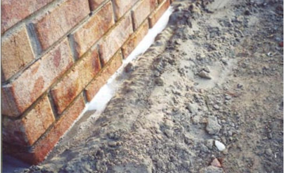
Chemical systems are normally used in conjunction with slab-on-ground construction. Traditional chemical treatments incorporate a chemical system under the slab and around the perimeter of the building.
