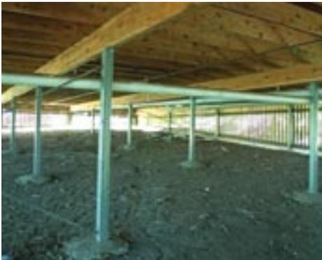
A minimum clearance of 400mm is generally necessary between the finished ground level, structural components and any other obstruction ( bearers, floor joists, plumbing pipes etc). The required clearance can be reduced from 400 mm to 150 mm provided the area slopes to and is not more than 2 metres from a point conforming with the required 400 mm minimum clearance.
