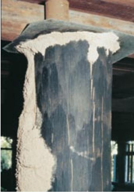
Until recently, physical systems have been restricted mainly to suspended floor construction (eg houses built on stumps). The traditional physical system is the ant cap. Ant caps are used primarily on elevated houses and are placed on the tops of stumps, piers etc. Ant caps will not prevent termites from getting into the building. They will act as a barrier to encourage the termites into the open where they can be noticed when inspections are carried out.
